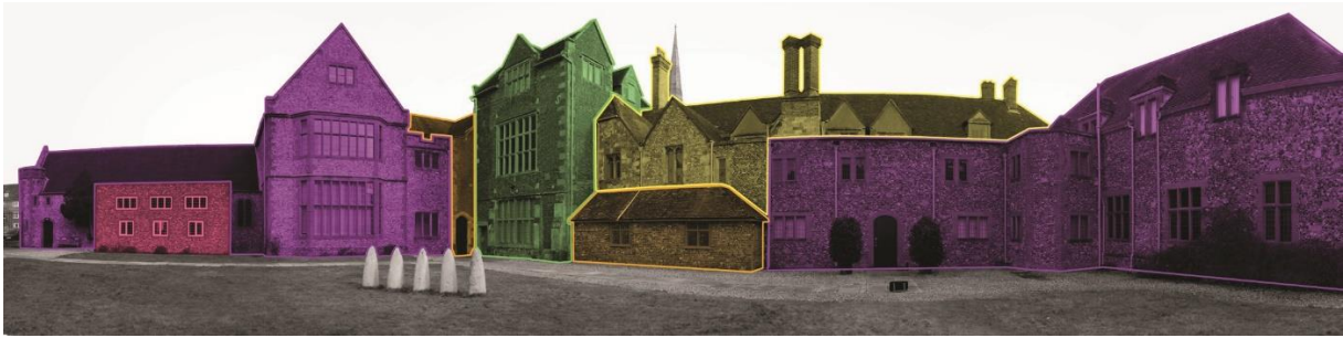
Rear of the King's House - different phases. See plan above for colour code
